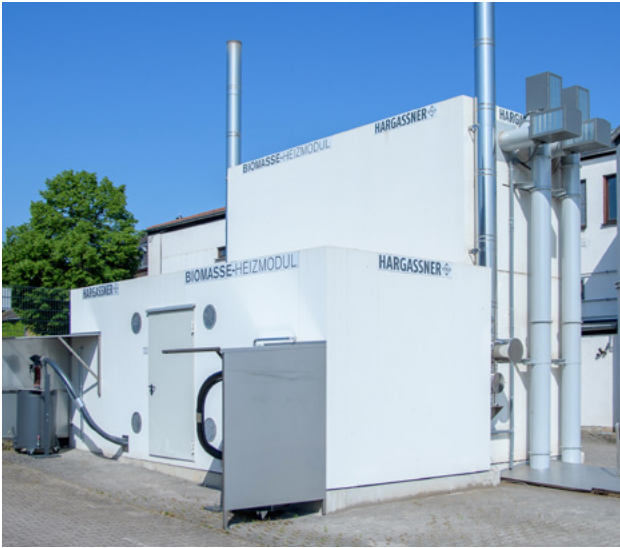
SIMO Fishprocessing in Merzig, 2 x 120 kW Hackgut
