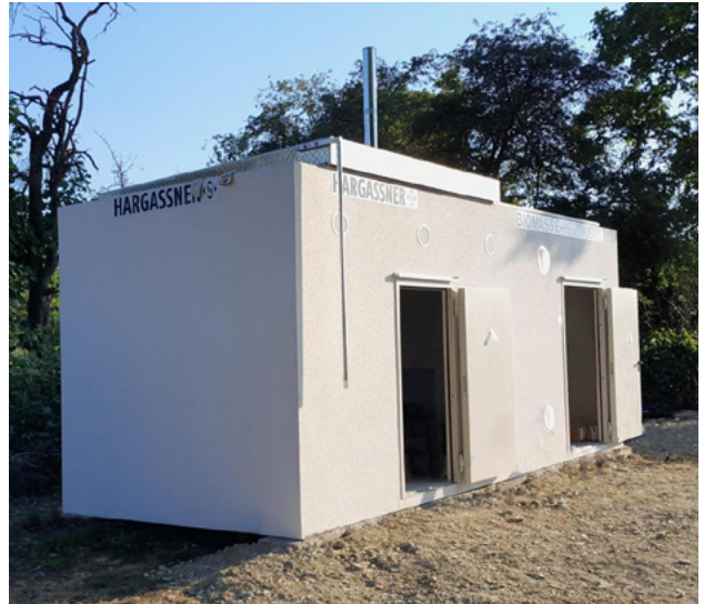
Sonrey in Dransfelden, 40 kW Hackgut
